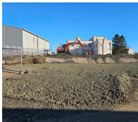
Extensive work to backfill the site followed the removal of all the soil.
