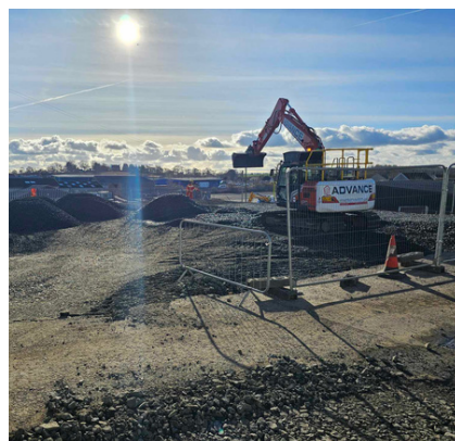
Extensive work to backfill the site followed the removal of all the soil.
